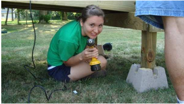
Clara drilling holes for a wheelchair ramp
