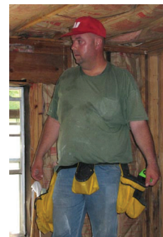
Mark Petersdorff in position to hang another piece of drywall
